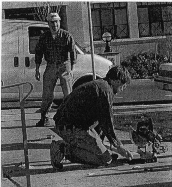
Jim Baskin and Don Winters Working On Forms For Front Patio
