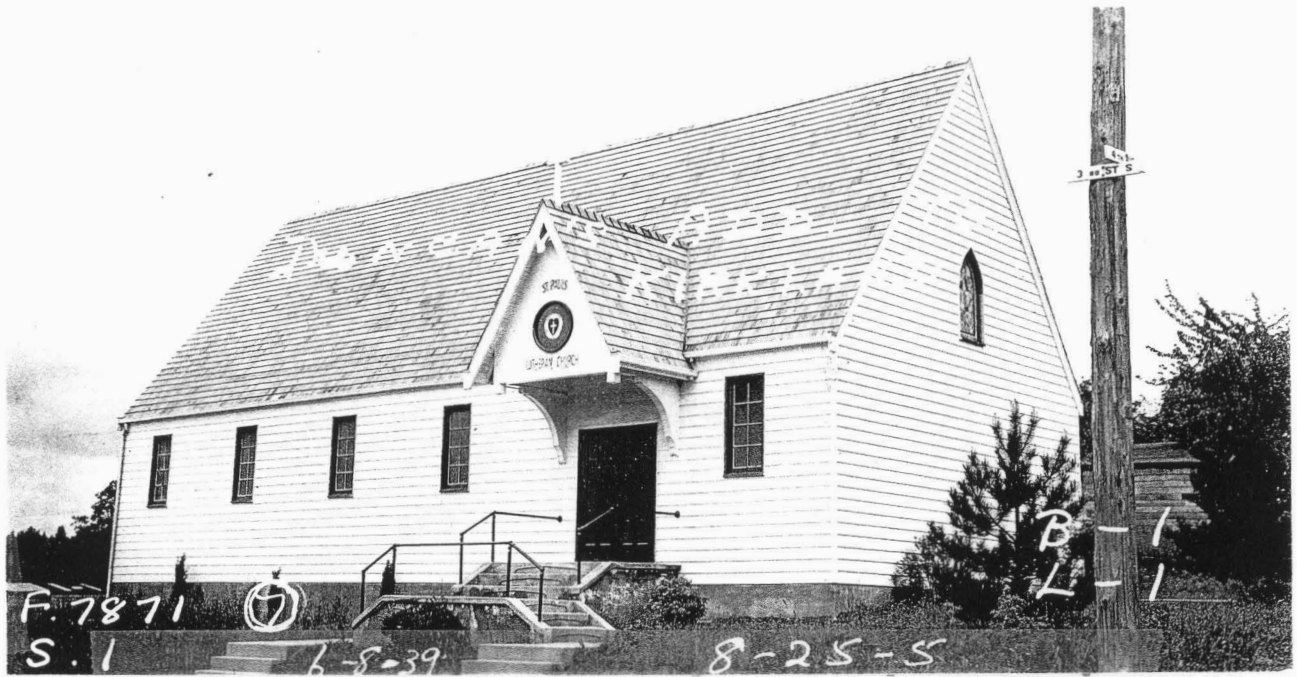
ST. PAUL'S LUTHERAN CHURCH - 1939 Assessor's Photograph from State Archives
